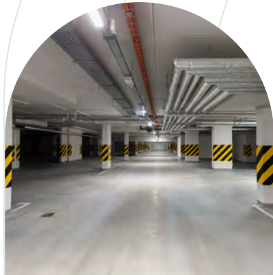
Spacious underground parking to avoid congestion.
